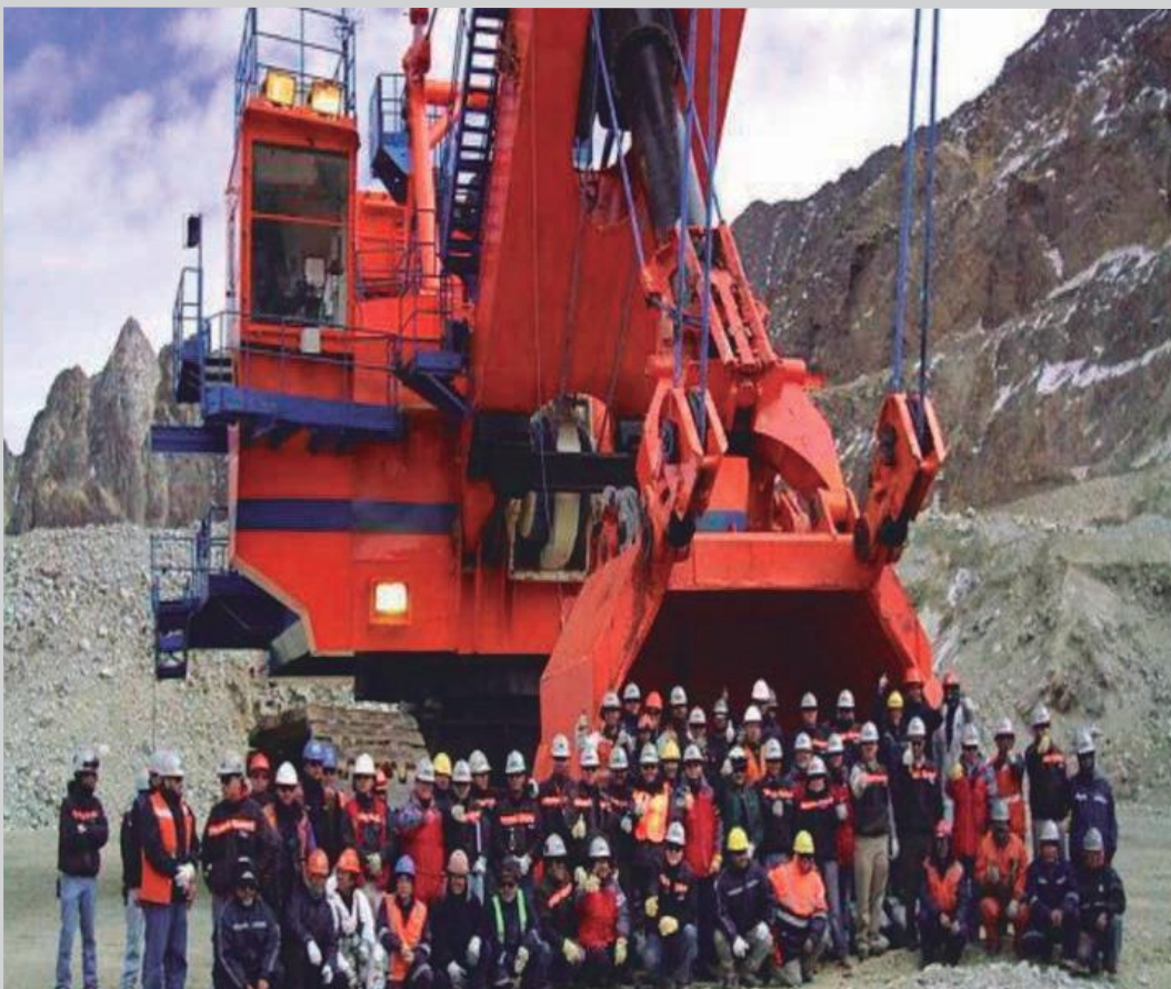
Overhaul, assembly, and commissioning of a Bucyrus Shovel at Los Bronces mine, Anglo American, Chile, performed by the MINETEC team.
